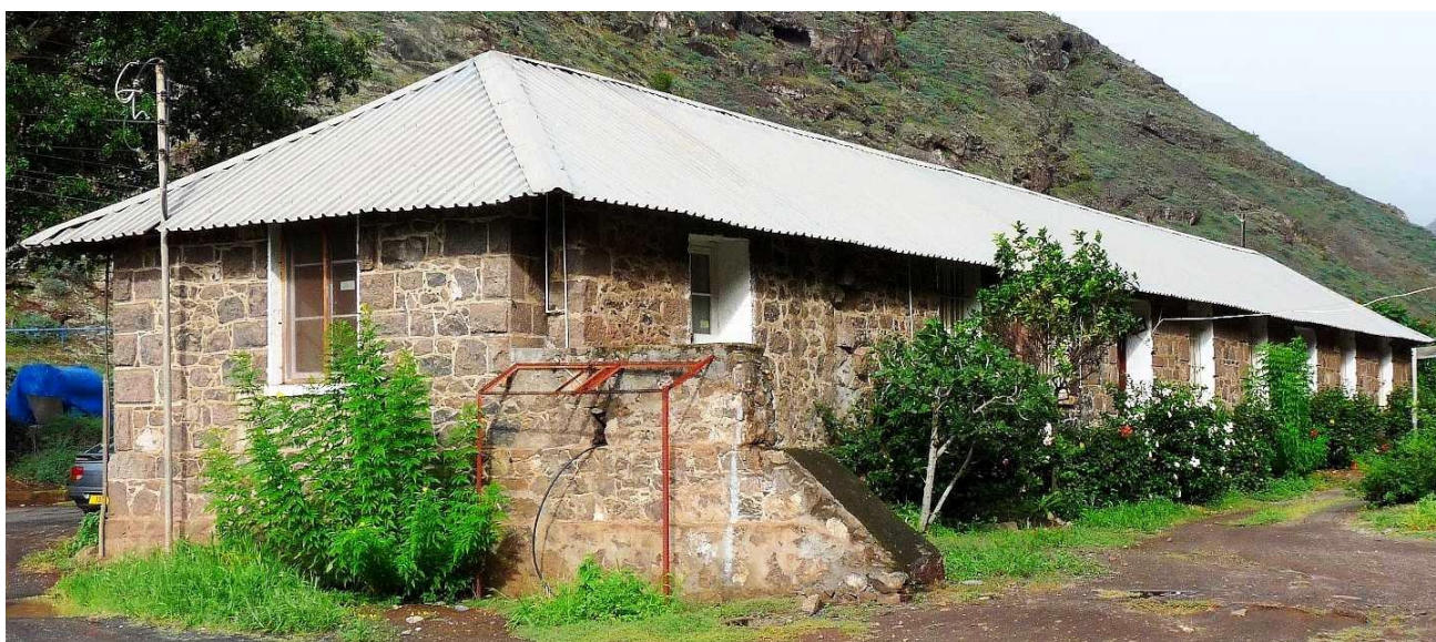
The No. 1 Building in Rupert's Valley, St Helena. Credit: St Helena National Trust
